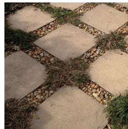
Pavers in gravel bed
