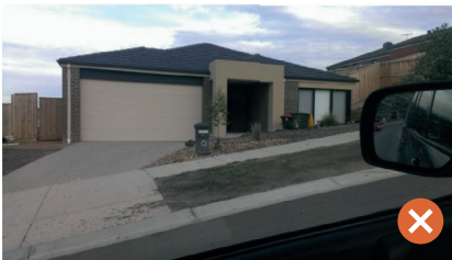
Flat pad on significant cross fall with no retaining
